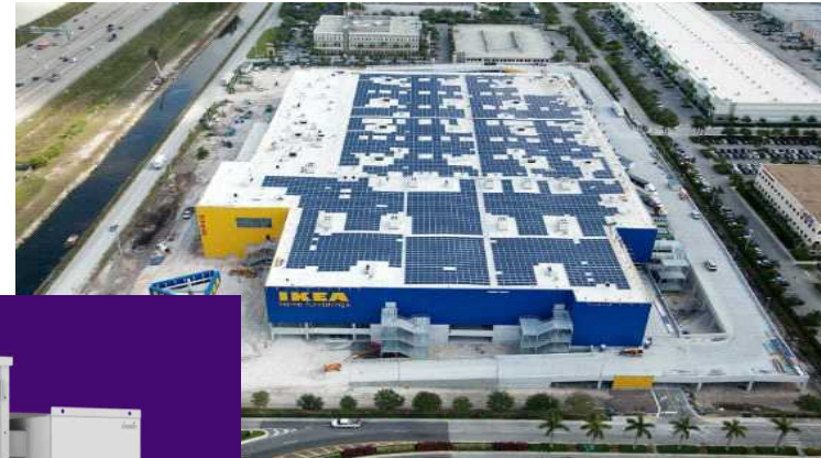
Net Zero Energy Building
